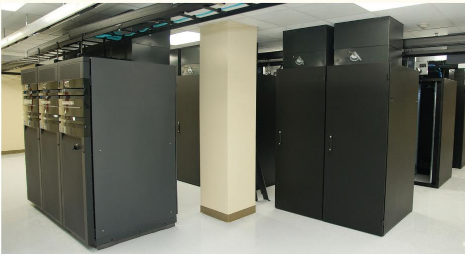
Gundersen's data center uses a chimney design to prevent hot and cold air from mixing, leading to energy efficiency and savings.
