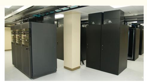
Gundersen's data center uses a chimney design to prevent hot and cold air from mixing, leading to energy efficiency and savings.
