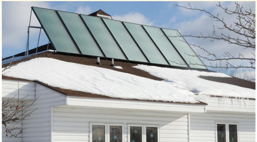
Gundersen installed solar panels on the roof of its Child Care Center as part of a solar hot water heater project. Fluid runs through the panels, gets heated by the sun and passes through a heat exchanger where the cold incoming water from the City heats up. The hot water is then ready for use in the building.
